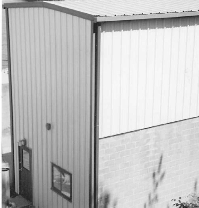
FIGURE 7.32 This partial-height CMU wall faces a hill and provides a measure of protection against rolling rocks and sliding debris.
